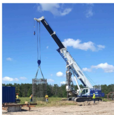
Foundation Installation
